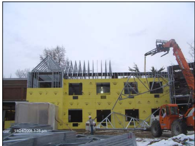
Roof trusses being put in place by crane.
